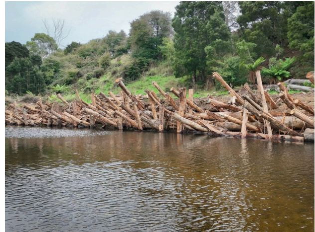
Inglis River Timber Revetments
